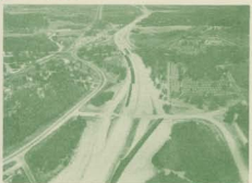
I-90-94 sweeps over County Trunk Highway "C" at interchange serving Camp Douglas, at left, and Camp Williams, at right.
